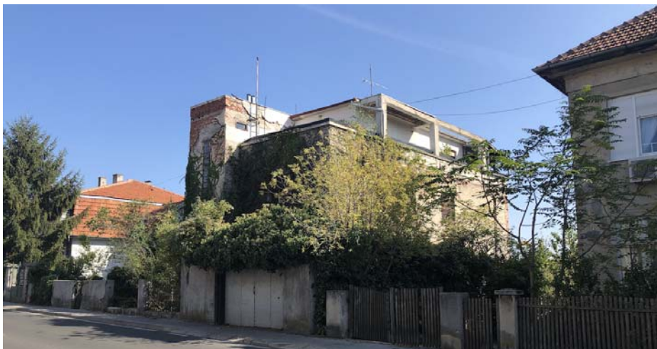
Figure 3. The photograph of the existing Mosinger Villa, view from the south-west (the Pantovčak Street) 2020.
