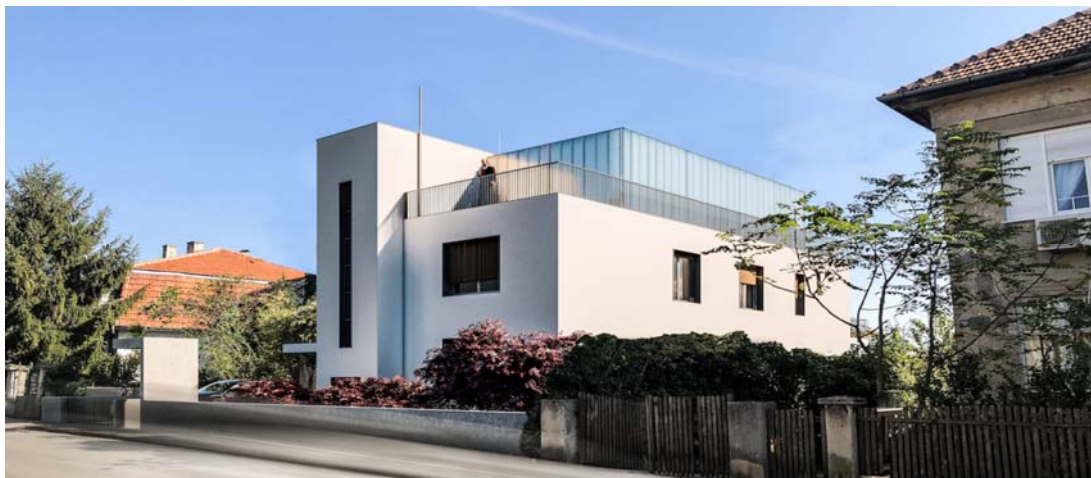
Figure 4. A 3D model of the future Mosinger Villa, view from the south-west (from the Pantovčak Street), 2022.
