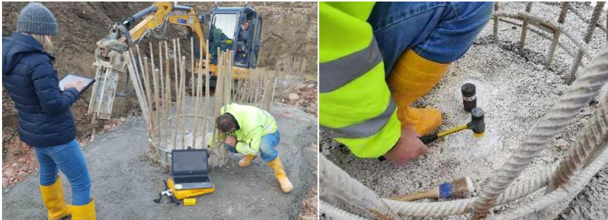
Figure 11. Testing the integrity of piles using the PET method (photos by authors)
