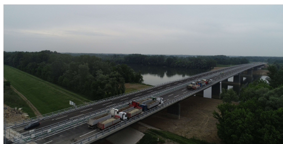
Figure 13. - Placing the load in position for static testing
