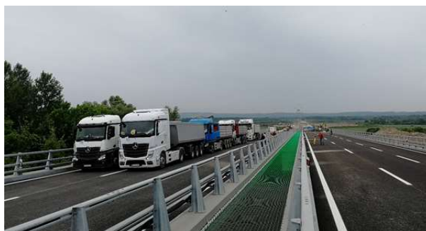
Figure 15. - Load in the position for static testing
