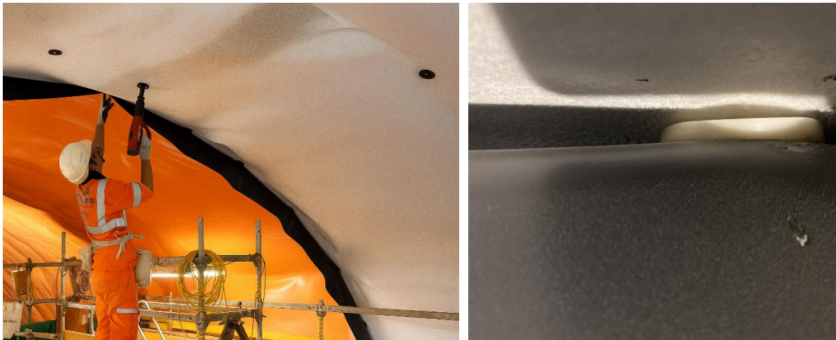
Figure 2. Illustration of the attachment of the protective felt and the waterproofing membrane [3]
