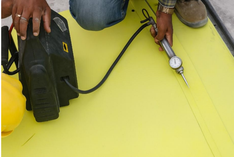
Figure 8. Testing of joints with compressed air [8]
