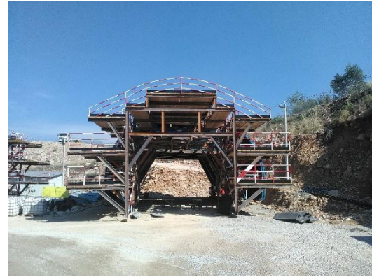
Figure 5. View of steel tunnel scaffolding, Vjeternik Tunnel, Montenegro [2]
