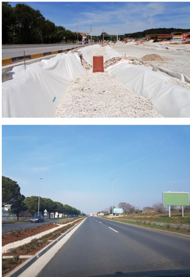
Figure 6. City bypass under construction and after planting (Starum) [10]
