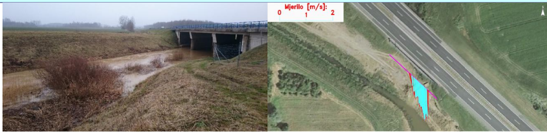
Figure 4. Lateral Channel: a) constriction of flow profile upstream from the bridge, view from the right bank (left); b) inverted flow velocity profile on orthophoto map (right)4
