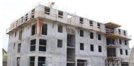
Figure 10. Prefabricated concrete system [17]
