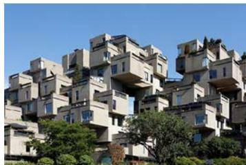
Figure 9. Prefabricated spatial system [16]
