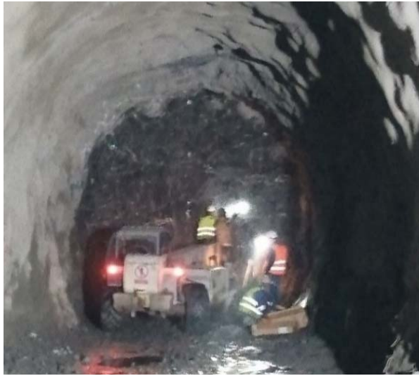
Figure 8. Filling of blast holes
