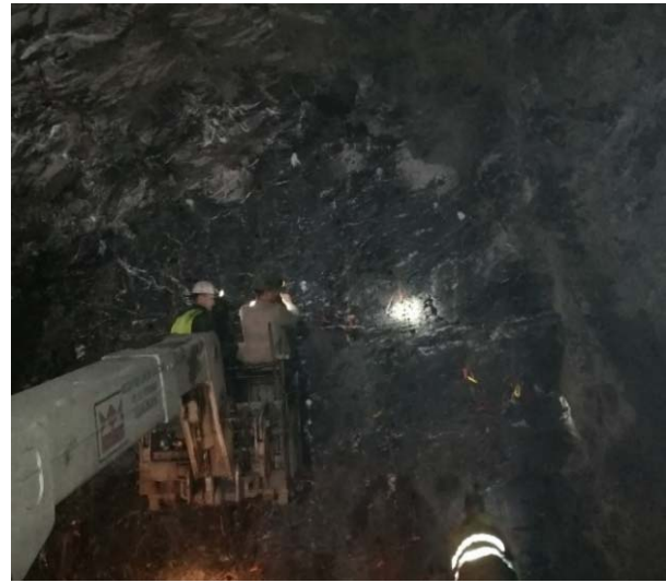
Figure 9. Connecting of blast holes
