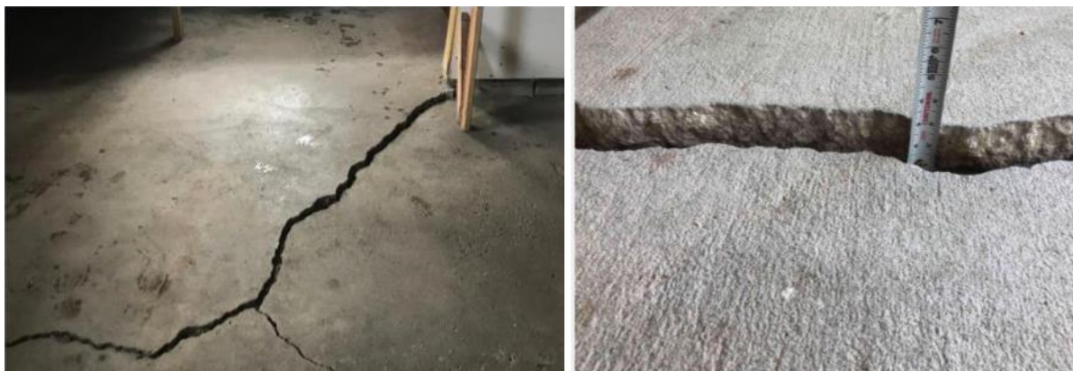
Figure 4. Cracks in a floor slab [5]
