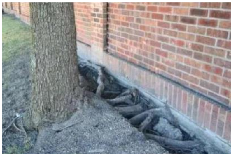
Figure 6. Cracks due to vegetation [6]
