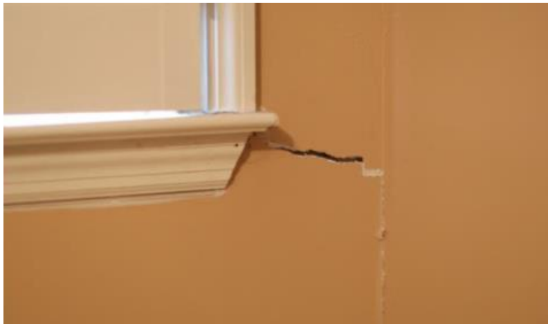
Figure 5. Cracks in walls [6]
