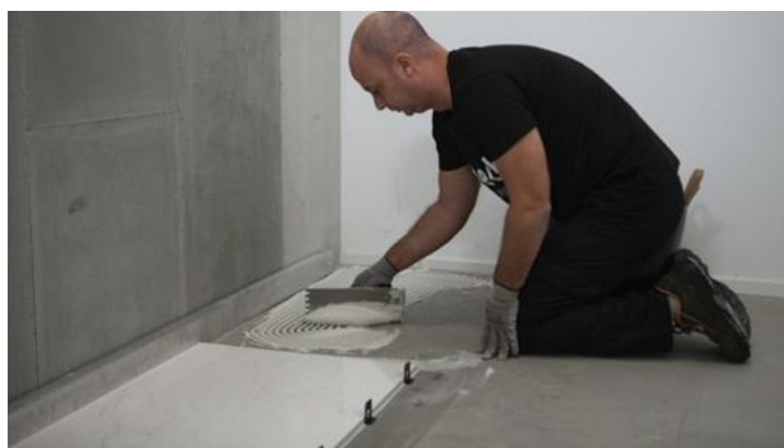
Figure 12. Tile installation process
