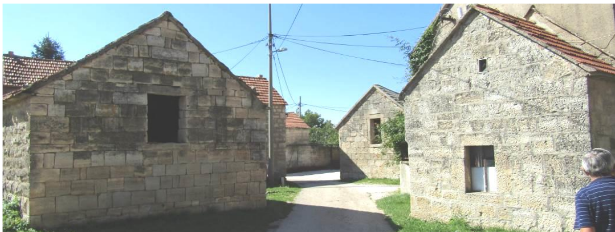
Figure 11. Relatively little patination of facades made of ( Posušje ) miljevina in Ramljaci-Čitluk near Posušje; Orientation of the building and its position in relation to the adjacent buildings are important, so there are certain differences when it comes to a standalone building, or a building that is the first/last in a row, (photo: K. Šaravanja), [21]
