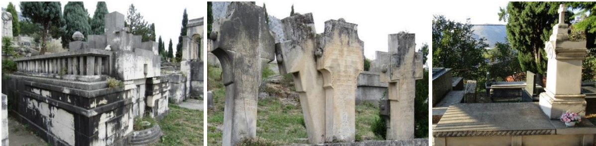
Figure 8-10. Different forms of patination and soiling of surfaces on tombs made of freshwater limestone in Mostar: Bjelušine cemetery (left and center); Although the grave crosses are almost of the same height and shape, they are patinated differently, which indicates not only their different age, but also probably the different quality of the stone, or different layers in the quarry from which they were extracted. The inscriptions on some of them have completely disappeared due to the action of rainwater or are difficult to read (middle); The contrast between the dark (horizontal) and light (vertical) stone surfaces of the tomb in the Šoinovac cemetery in Mostar, along with the patinated inclined and smaller horizontal surfaces of the tombstone, create the impression that the tomb made of (Mostar) miljevina was made of several types of carbonate lithotypes (right), (photo: K. Šaravanja), [21]
