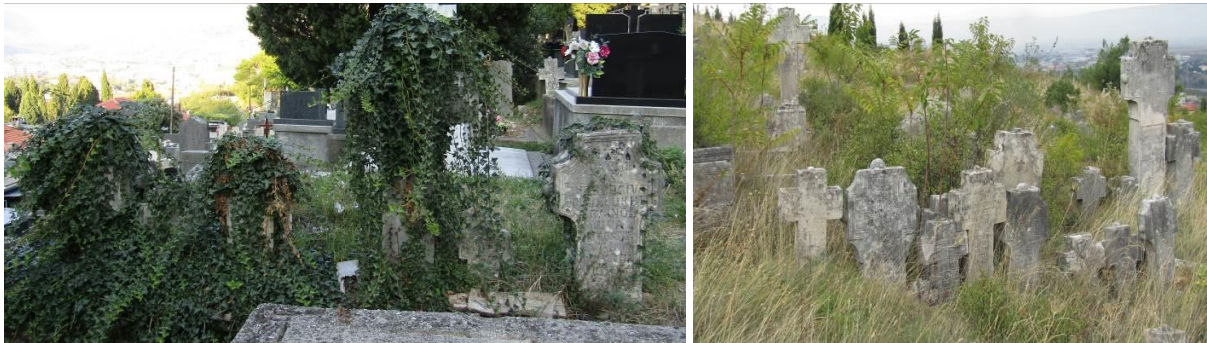
Figures 38-39. Ivy vegetation as an example of biological covering of tombstones in Šoinovac cemetery in Mostar (left); Tombstones in the old part of the Bjelušine cemetery in Mostar (right), which is neglected and overgrown with low wild vegetation, and a large number of monuments are overgrown with lichen and moss. During the war, all tall vegetation was removed from the cemetery area, which to a certain extent had previously protected the monuments from the sun and western winter winds, (photo: K. Šaravanja), [21]
