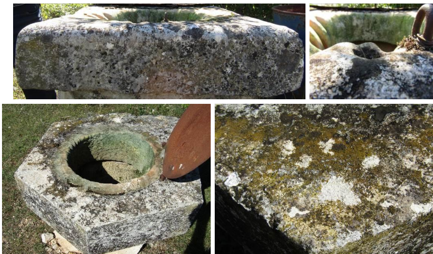
Figures 48-51. The crowns of stone cisterns made of (Posušje) miljevina covered with lichen and moss at the location of the Kovači hamlet, southwest of Posušje, with details, (photo: K. Šaravanja), [21]
