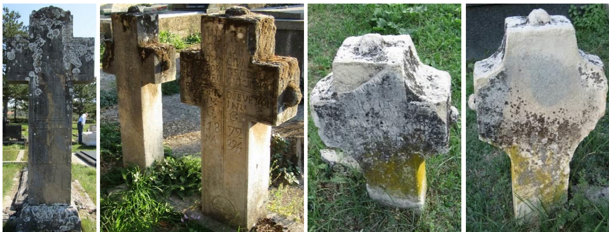
Figures 40-43. Covering of tombstones made of miljevina with biological cover in the cemetery of St. Ivo in Livno (left) and in the Šoinovac cemetery in Mostar (other 3 figures); Biological covering (lichens, moss, fungi,...) use stone as habitat and/or food, (photo: K. Šaravanja), [21]
