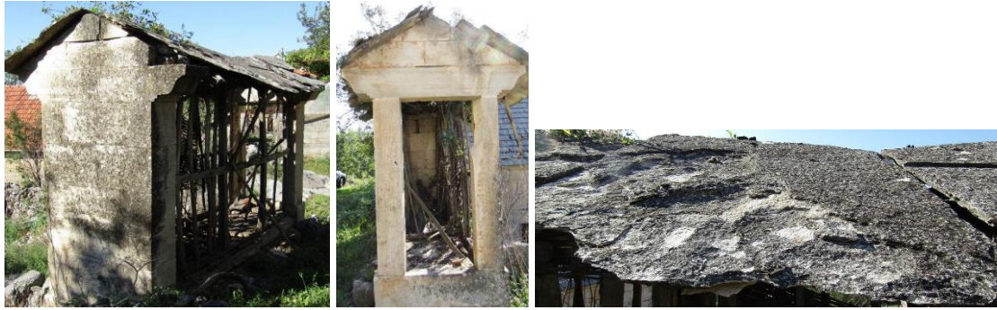
Figures 12-14. Corn storage (corn crib) in Tomić Brig near Posušje, about 120 years old, with dimensions 3x1.5 m; one can see the excellent preservation of the (Posušje) miljevina stone, especially the entrance part, which has less patina (middle); A cover made of stone slabs 0.2-0.3 m 2 in area, about 3 cm thick, covered with patina, with some lichen (right) deserves special attention, (photo: K. Šaravanja), [21]
