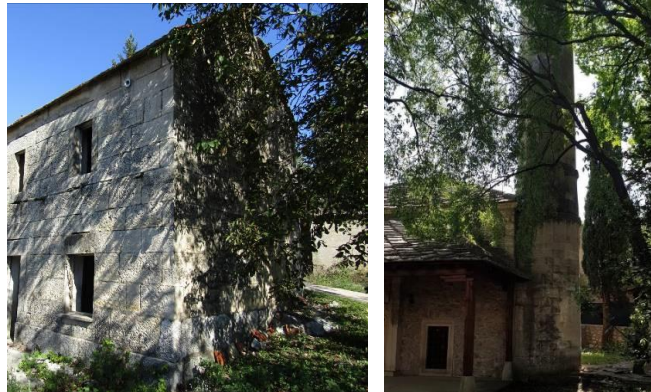
Figures 13-14. Examples of the influence of the surrounding vegetation: a house in Tomića Brig-Vinjani near Posušje, with the influence of the nearby walnut tree on the east side of the building, whose leaves, when washed by rain, acidify the rainwater to some extent (left); The minaret of the mosque near the Bunur pedestrian bridge in Mostar with a more intense patination of the stone due to the proximity of the surrounding vegetation and the Neretva River (right), (photo: K. Šaravanja), [6]
